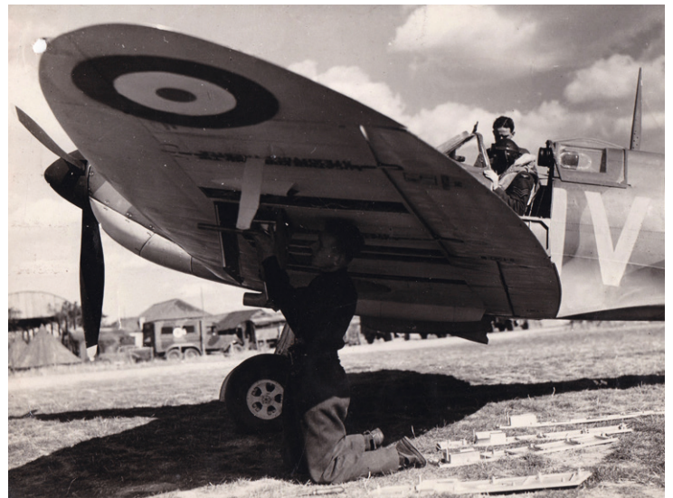
Late production Spitfire Mk.Ia, with full armor including windshield armor, GM2 gun sight, gun-heating (with gun heating firings on the bottom side of the wing), late style antenna mast and Pitot tube, De Havilland 5/20 propeller, rear mirror and voltage regulator behind the headrest.
